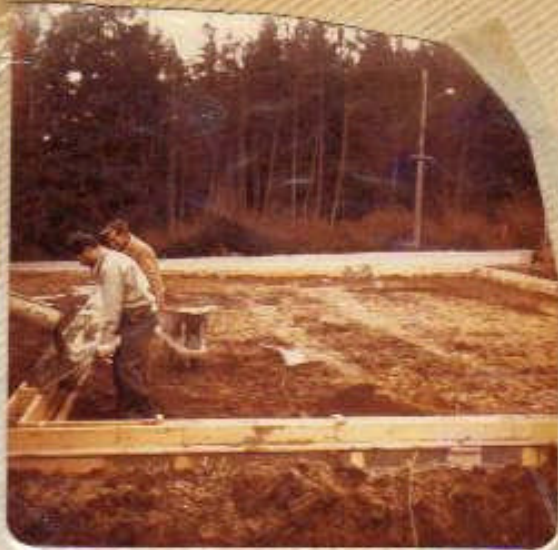
MERRITT & TED MAXWELL BUILDING FORMS FOUNDATION
